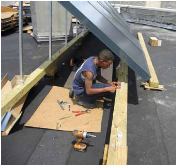
A worker installs a thermal solar system in New York City.
